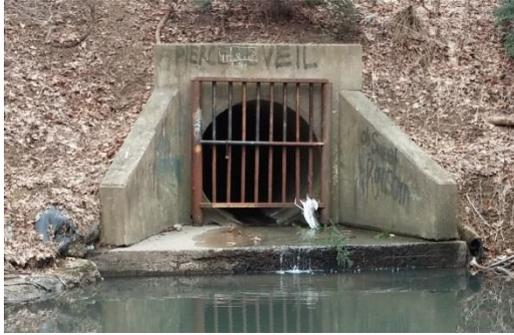
The other system, and the one we don't spend any money on, is the stormwater sewer system that conveys rainwater from the Borough. Stormwater runoff flows to one of our 577 catch basins in the street, is conveyed through the carrier pipes to one of 5 outfalls. Only one of the outfalls is actually to a creek, that being the outfall behind Beggs Snyder Park.
